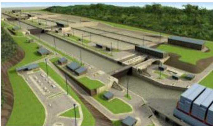
Figure 4: Conceptual view of finished Third Set of Locks for the Panama Canal
