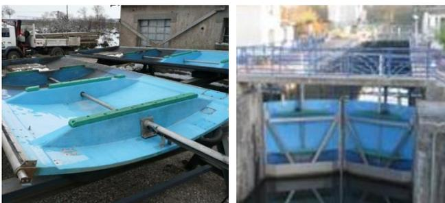
Figure 4: Goleby Lock, France. Supporting metal frames on the down stream side of the Gates.
