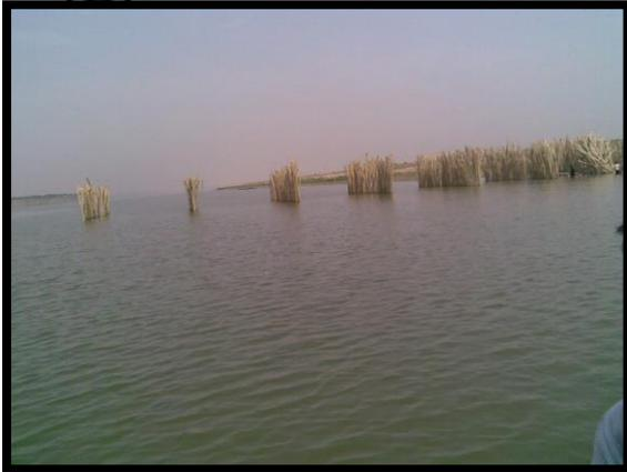
Figure 2(A): Bamboo Submerged Vane on Ganga for secondary channel closure
