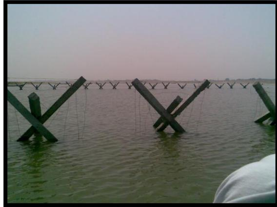
Fig.2(B): RCC Jack Jetty Screen on Ganga for secondary channel closure
