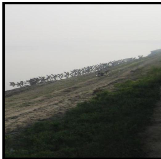
Figure 2 (E): Silting And Erosion Control with the RCC Jack Jetties on Ganga river
