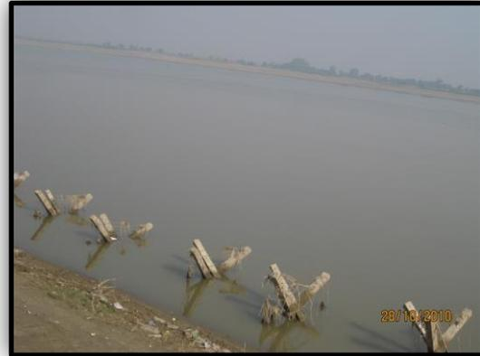
Figure 2(D): RCC Jack Jetty diversion line on Ganga for erosion control
