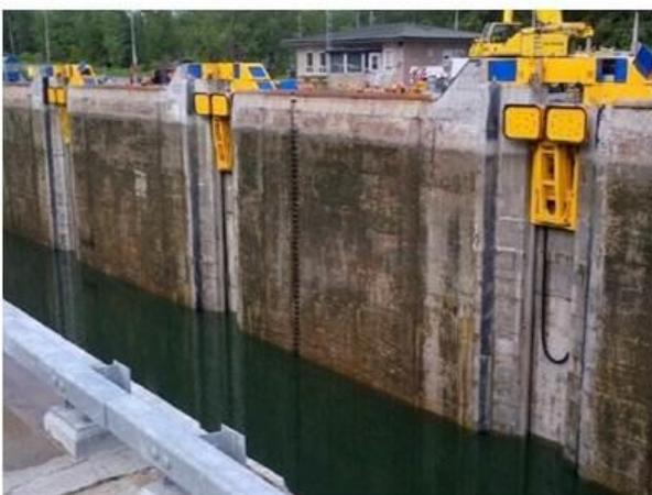
Figure 4: Three double units recessed in a lock wall
